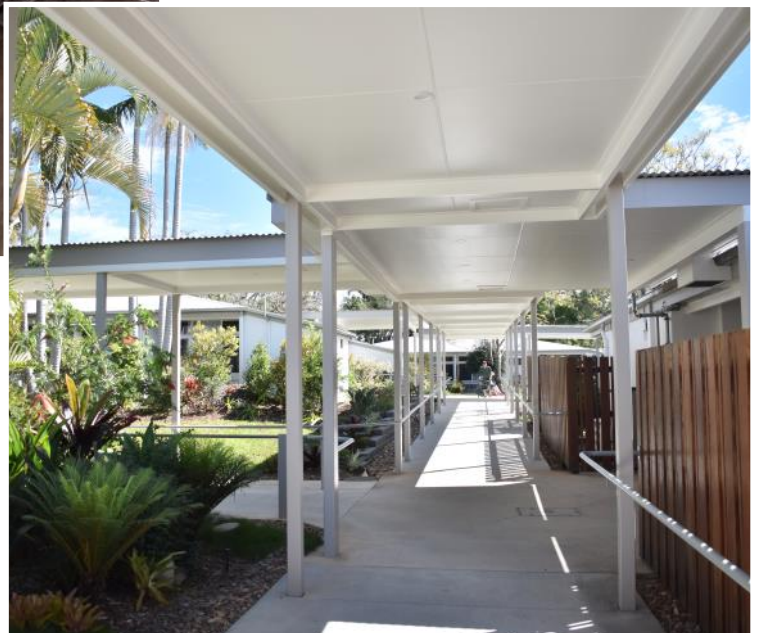
Walkways project completed at Carramar
